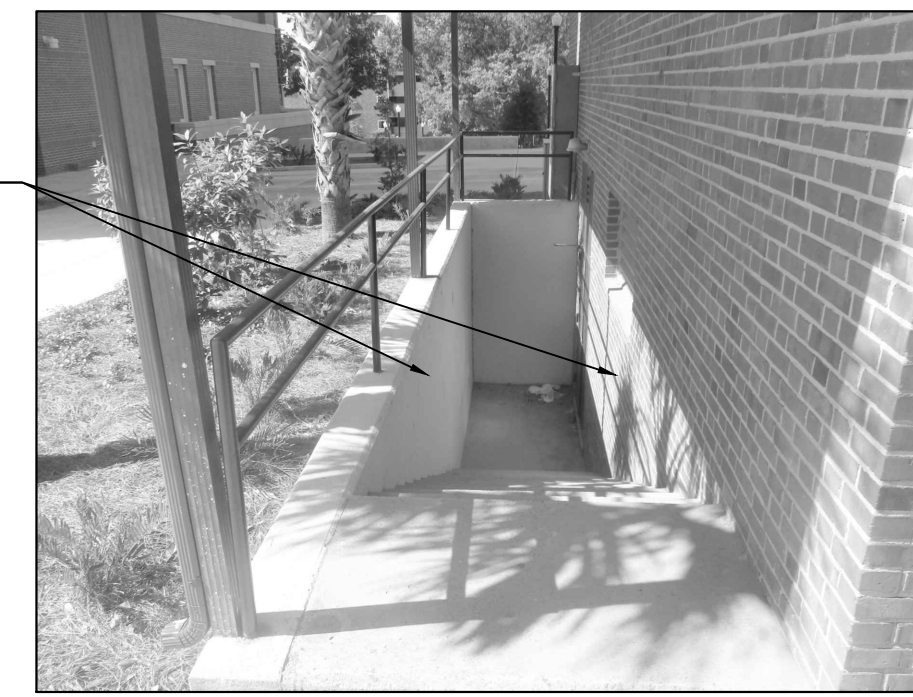
B VIEW OF STAIR OUT OF COMPUTER SCIENCE MAJORS LABORATORY 025
