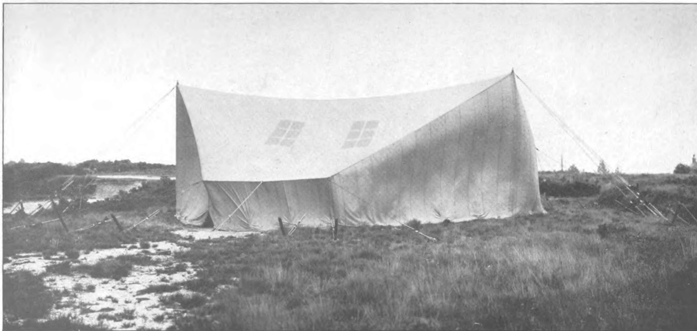
FIELD TENT FOR AEROPLANE: BACK VIEW. Supported by two poles only ; Roof ridge formed by stretched wire rope. Designed R.A.F. 1913.
